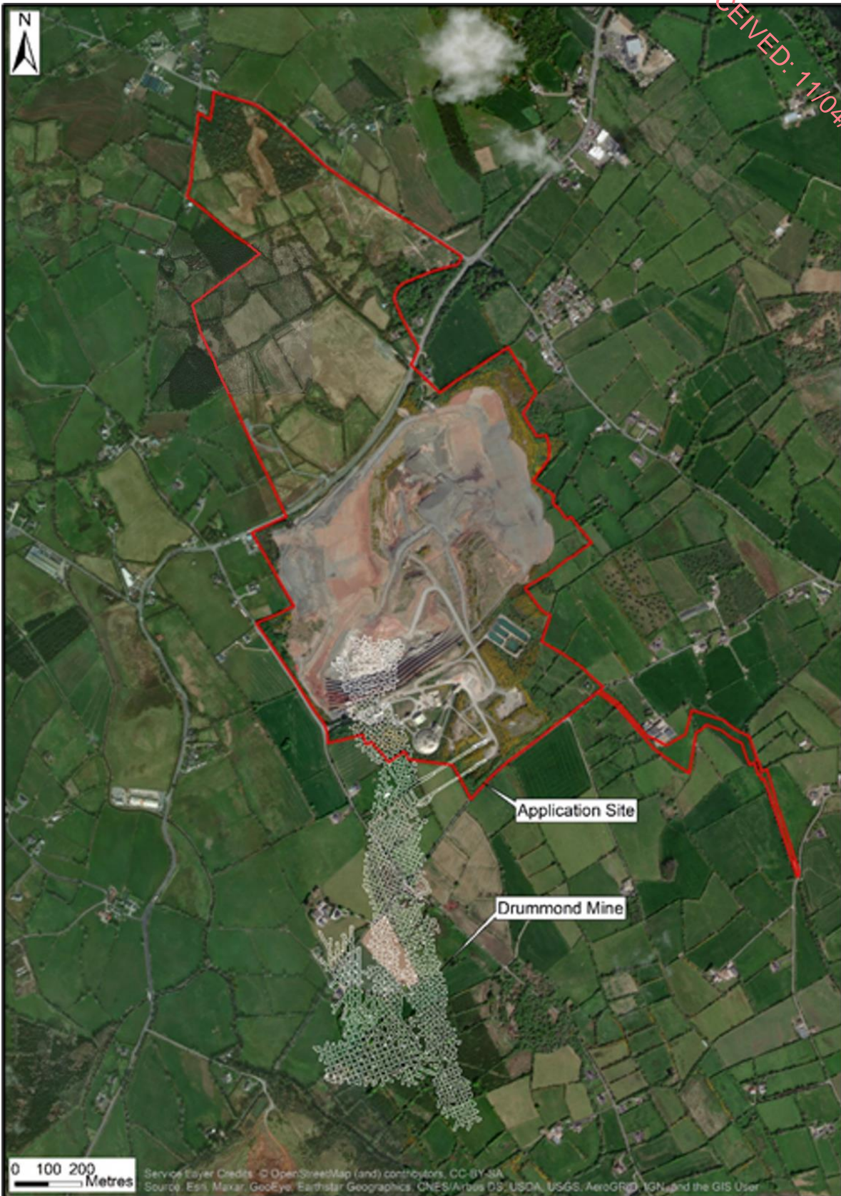
Figure 1.2: Drummond Mine Area (30 September 2021)
