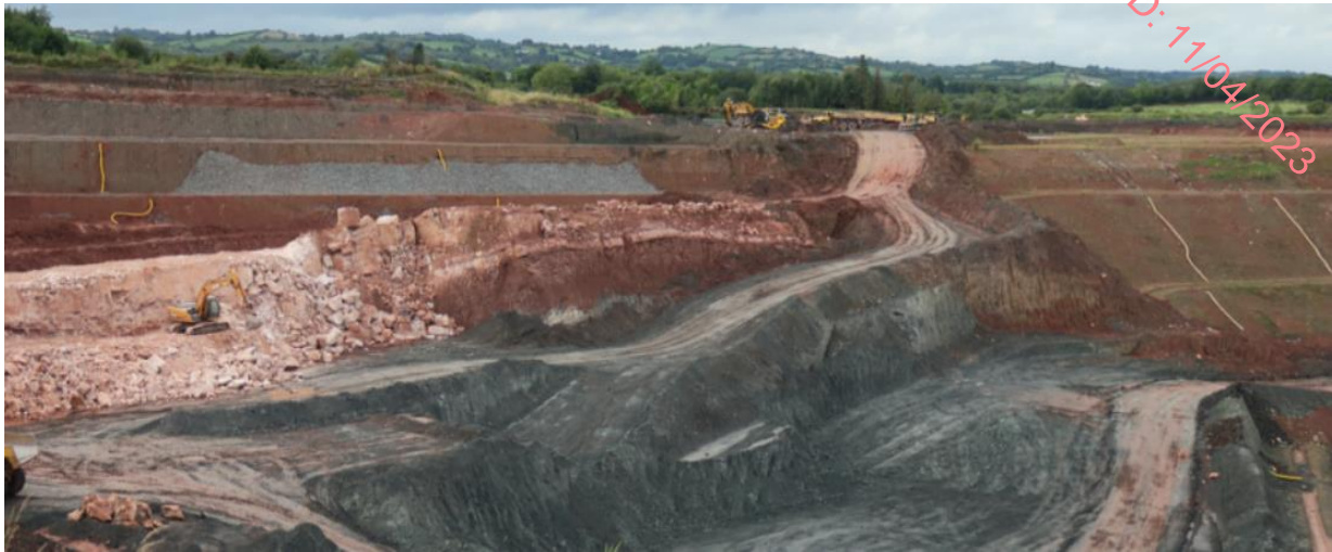
Figure 4.2: Good surface runoff management practices at the Knocknacran open cast, including plating of the bench faces and drainage of the benches
